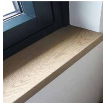
WINDOW drywall wrap with wood sill
