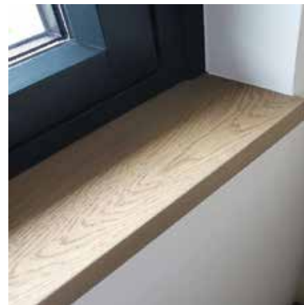
WINDOW drywall wrap with wood sill
